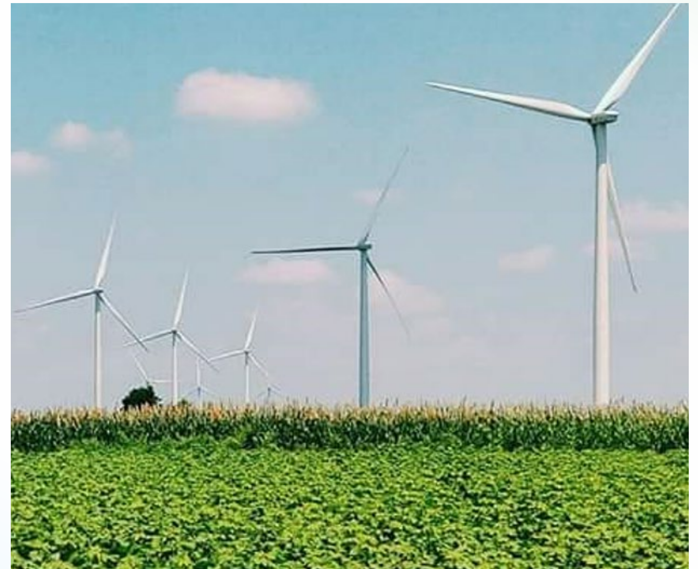
Windmills installed in Andhra Pradesh by a SBI financed group.
