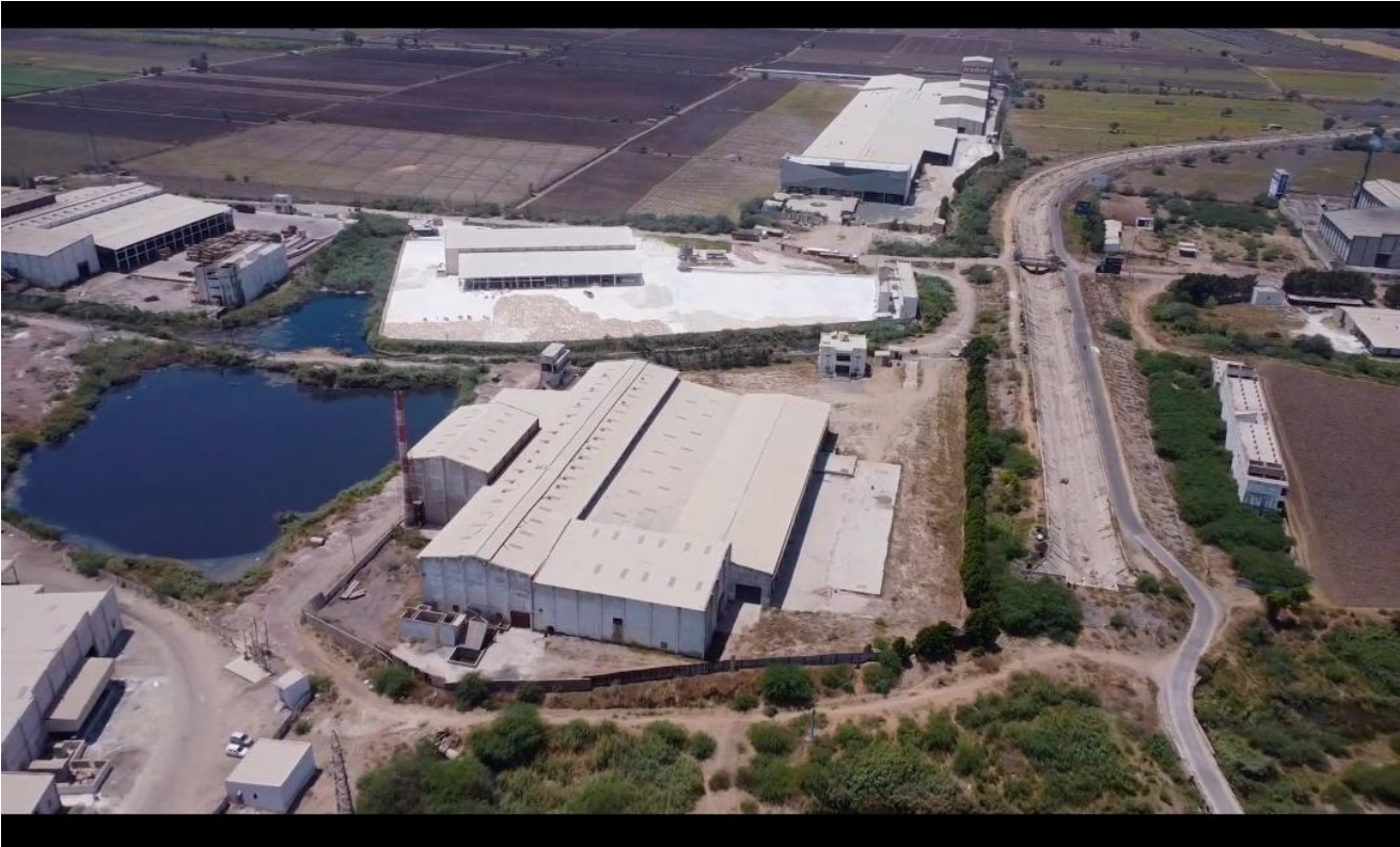
Factory Land and Building at Kerala Vi Morbi:
